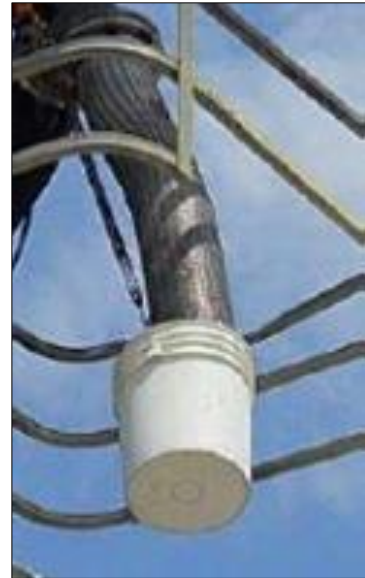
Figure 18: Use of Bucket to Reduce Spillage
