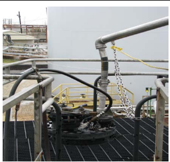
Image 23: Loading arm secured to siphon pipe
