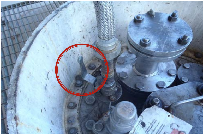
Image 21: Top fittings with flange assembly as alternative to siphon pipe cap
