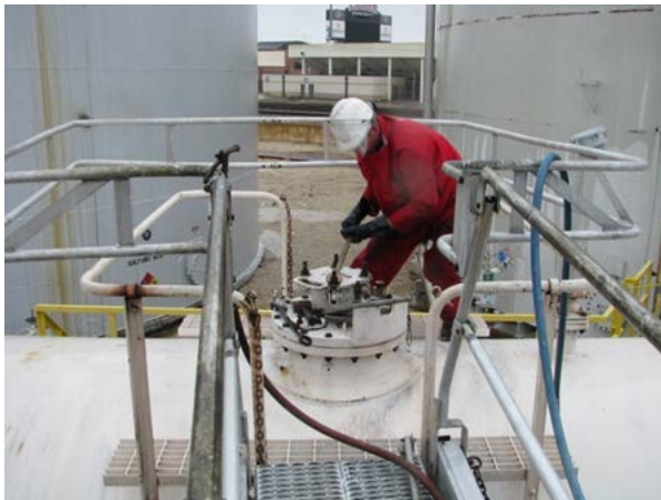
Image 2: Operator using open-ended wrench to achieve a tool tight condition
