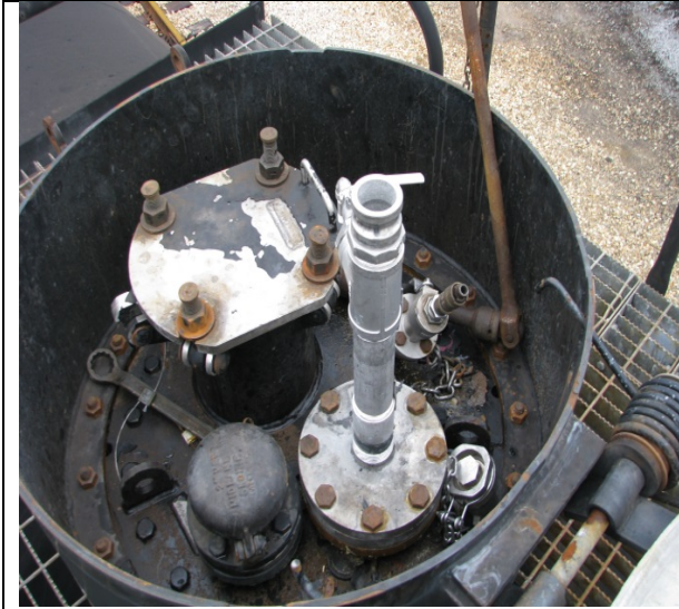
Image 22: Siphon pipe secured to tank car
