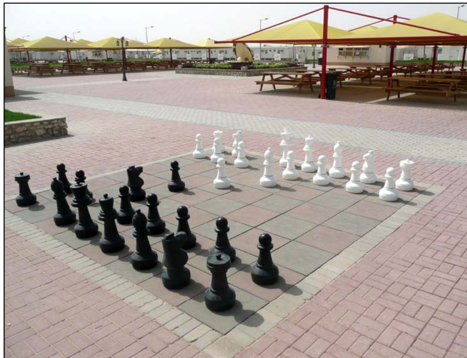
Figure 7: Shell sulphur concrete chessboard after installation.
