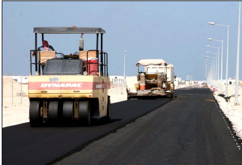
Figure 10: Sulphur-modified asphalt mix laydown in RLIC, October 2007.
