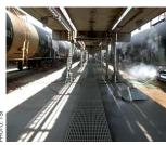
Steam feeds to liquid sulphur rail cars.
